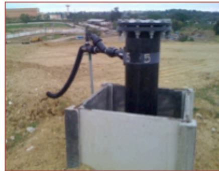
2. Biogas capturing well installed.
