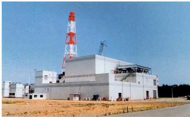
Figure 3: View of the reactor HTTR [6].
