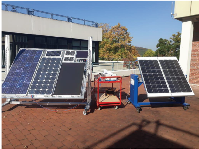
Figure 15: PV Modules installation for outdoor measurements.
