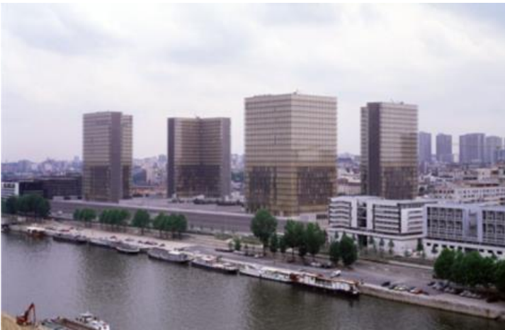
Figure 12: National Library, Dominique Perrault [39].
