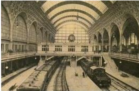
Figure 3: D'Orsay Railway Station [25].
