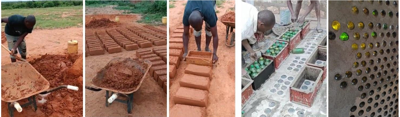
Figure 4: Adobe construction technique using locally available earth about 50 meters from the construction site and bricks or walls made by reusing plastic or glass bottles and raw earth or cement.
