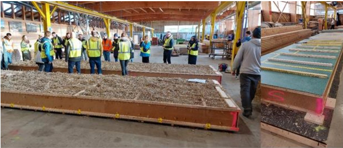
Figure 11: Showing straw bale modular wall system in manufacture with straw bale installation LHS and complete panel RHS. Chênelet northern France [Source Author].
