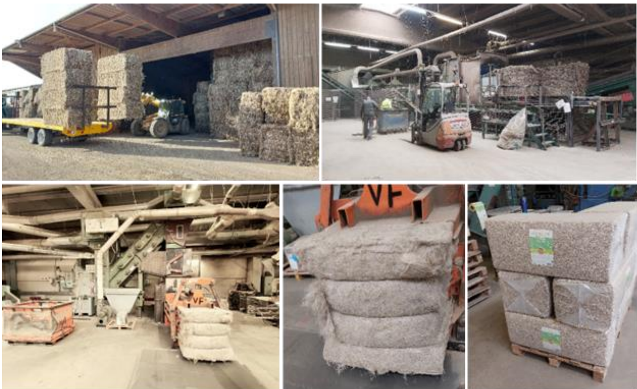
Figure 14: Hemp processing facility showing hemp bales input/storage, hemp processing and fibre/shiv outputs. Planet Chanvre Northern France [Source Authors].
