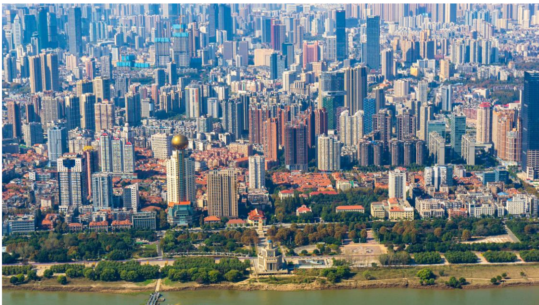
Figure 1: The Generic City in Asian metropolises - Image showing high-density heterogeneous central urban areas in Wuhan City, China (VCG.COM, with permission for academic publication).
