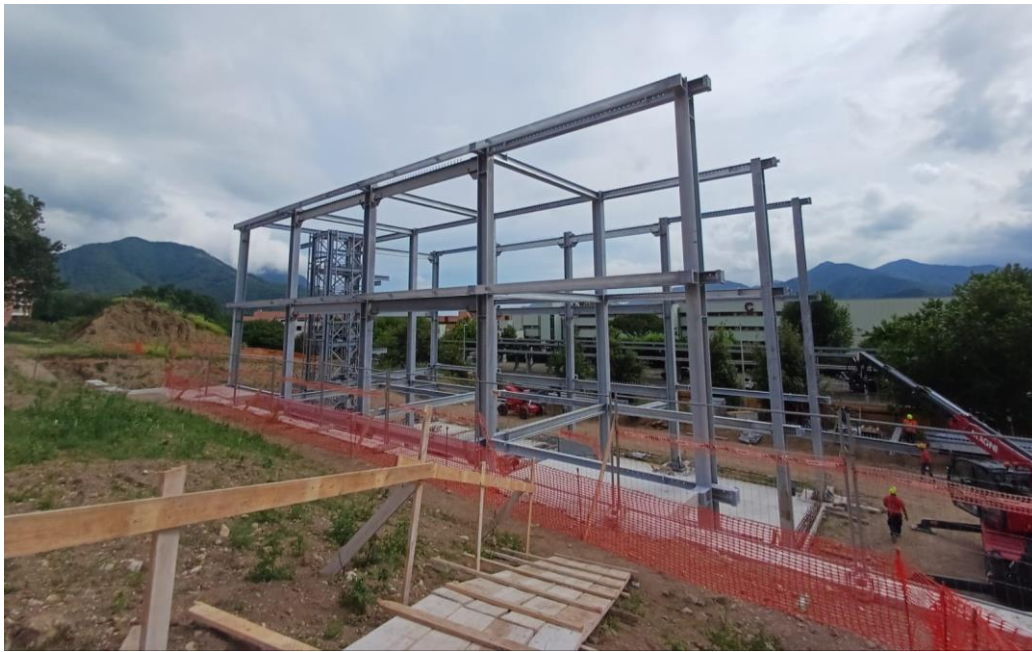
Figure 7: Steel load-bearing structure.
