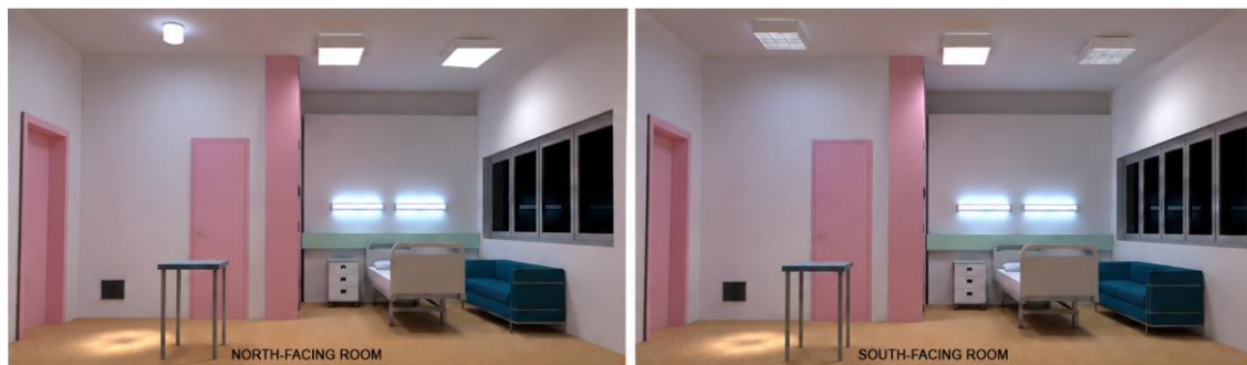
Figure 4: Existing artificial lighting arrangement in the north- and south-facing patient rooms: ceiling luminaires, bedhead lighting units, and low-level night lighting.
