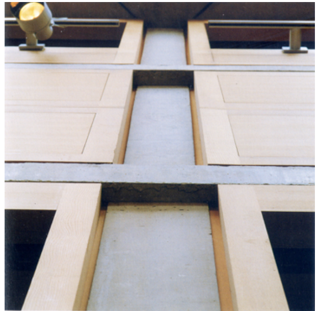
Figure 10: Inward inversion of the supporting columns. (Source: Wiseman, C. (2007), Louis I. Kahn: Beyond time and style, New York: W. W. Norton and Company Inc., 249).
