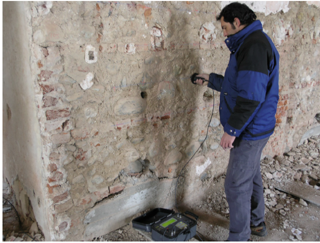
Figure 5: Sonic tests carried out at the Royal Palace of Venaria.
