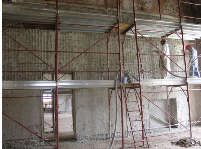
Figure 8: Jacketing wall technique made in the Royal palace of Venaria.
