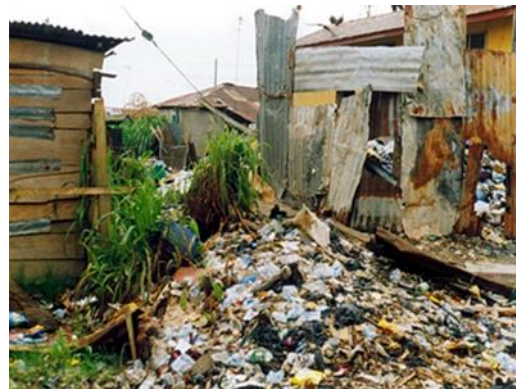
Figure 9: Backwater channel blocked by solid waste (Source: Ebakpa 2018).
