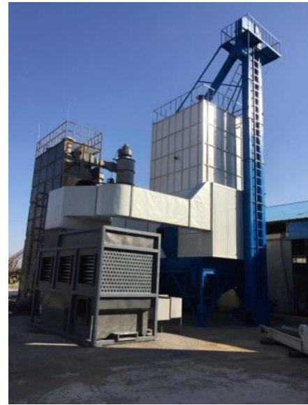
(2) Internal photo of drying system
