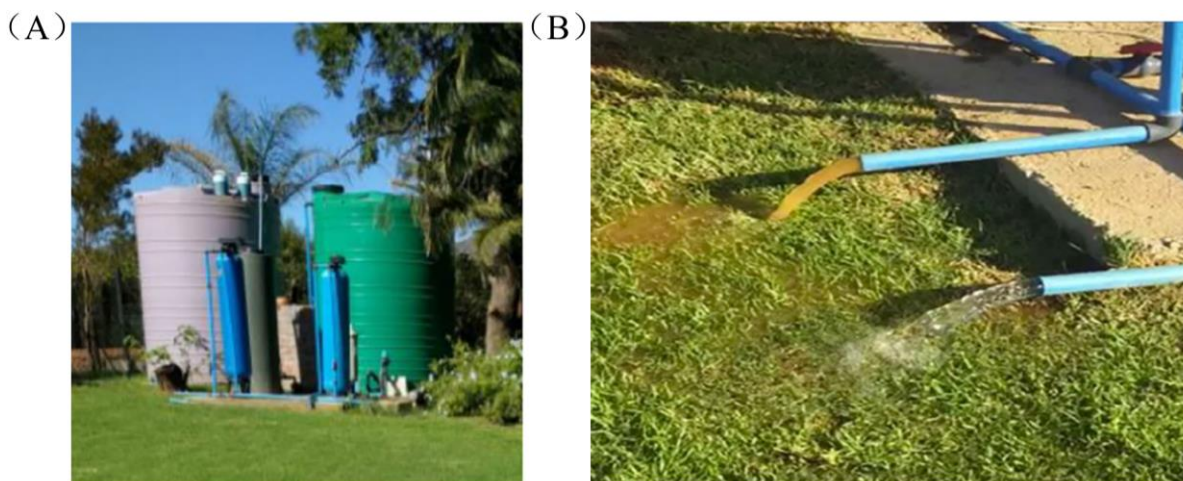
Figure 4: (A) Raw water tank, treated water tank, sand filters, and MK3 nanobubble generator + ozone generator and (B) visual characteristics of raw and treated borehole water [91].
